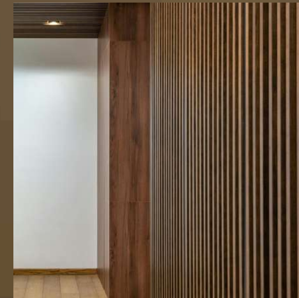
False Ceiling & Light Partitions Installation
