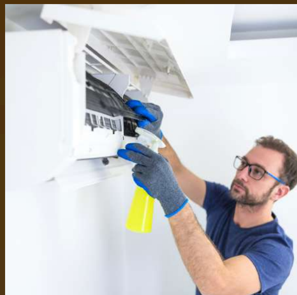
Air Conditioning, Ventilation & Air Filtration System Installation & Maintenance
